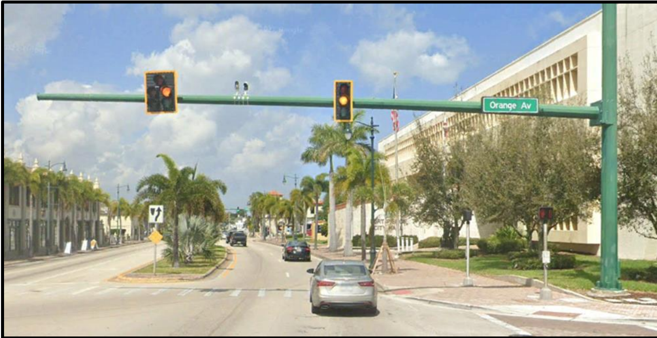
Traffic signal backplate installations for increased visibility of signal lights
