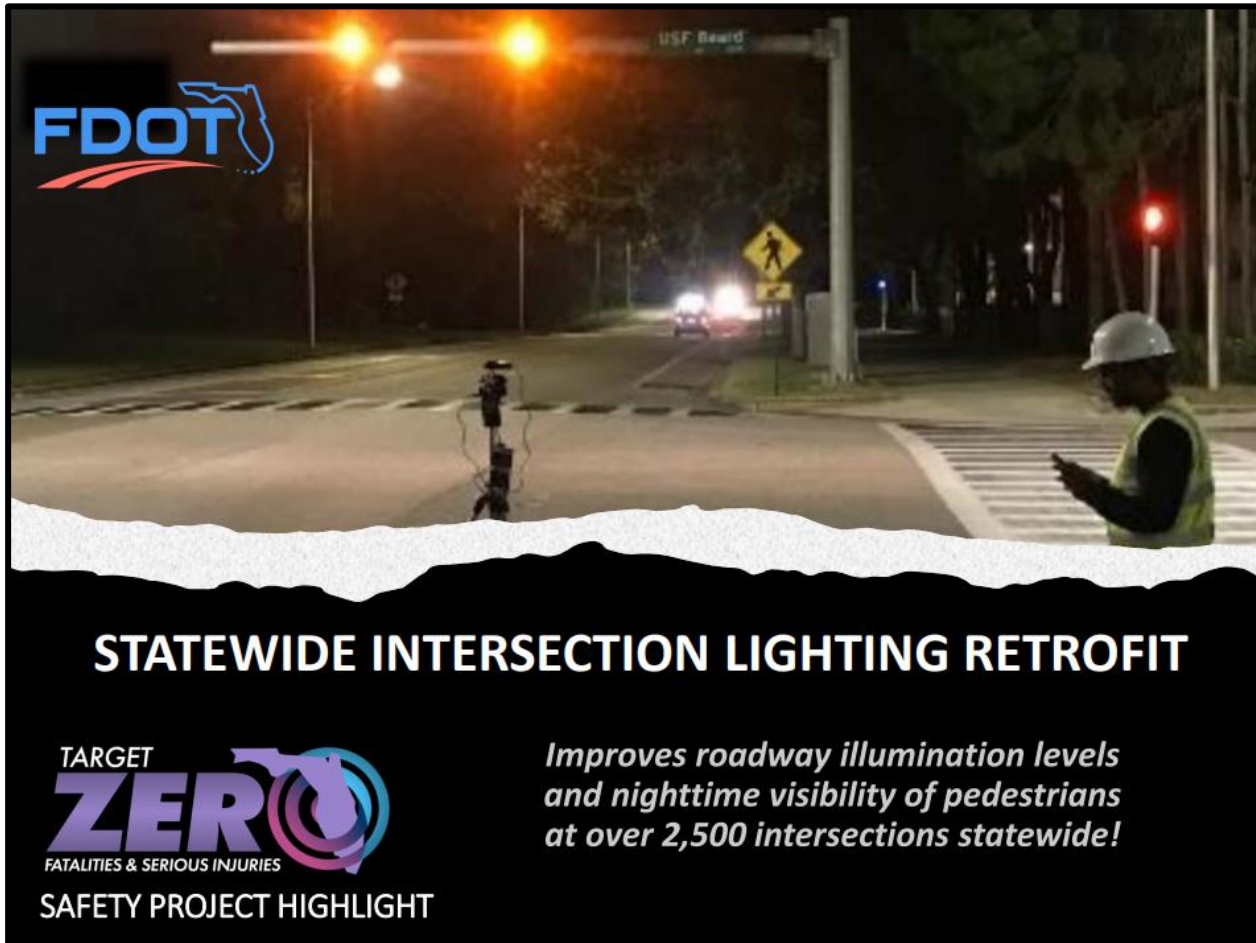
Retrofitting pedestrian lighting at signalized intersections
